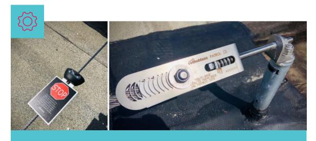
Horizontal Lifelines – like all height safety equipment – should be visually inspected immediately before and after use.
