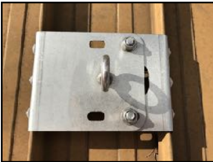
Surface mounted anchor
